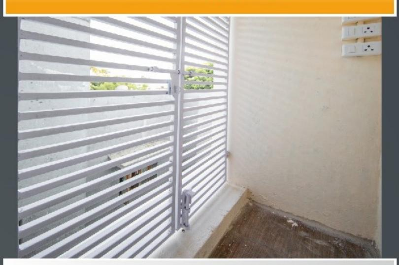
No exposed Out door Ac units with access through shaft doors - Enhances Iconic elevation
